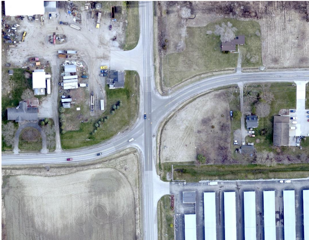
Figure 10: Aerial view of Lennon Road and Elms Road
