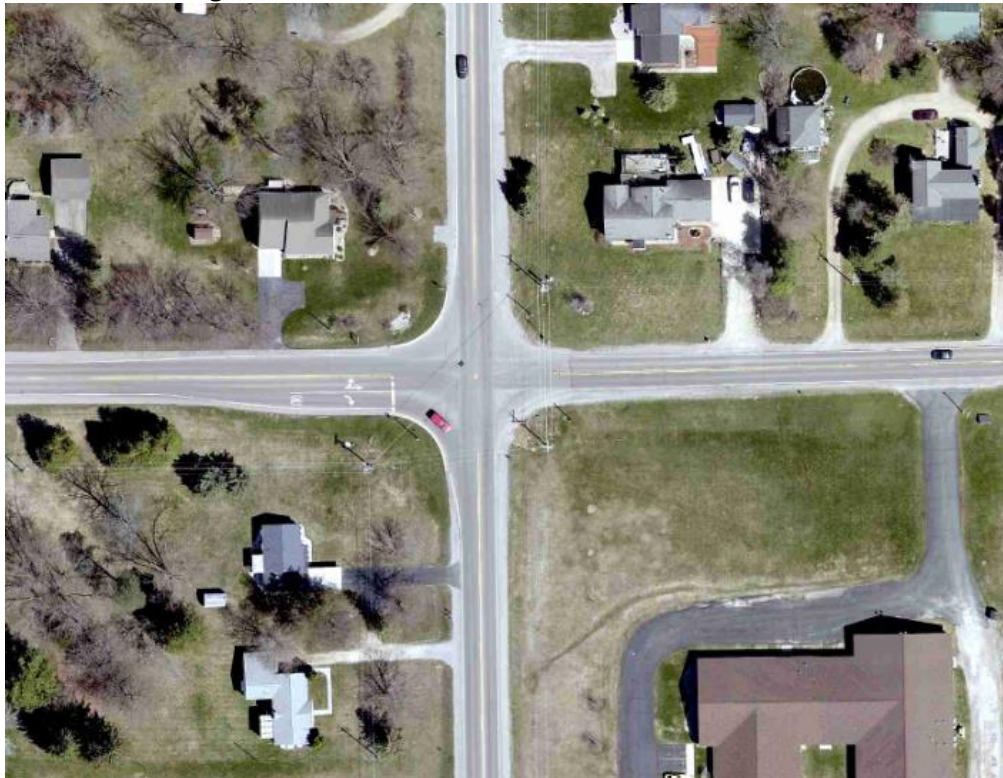
Figure 6: Aerial view of Coutant Road and Elms Road
