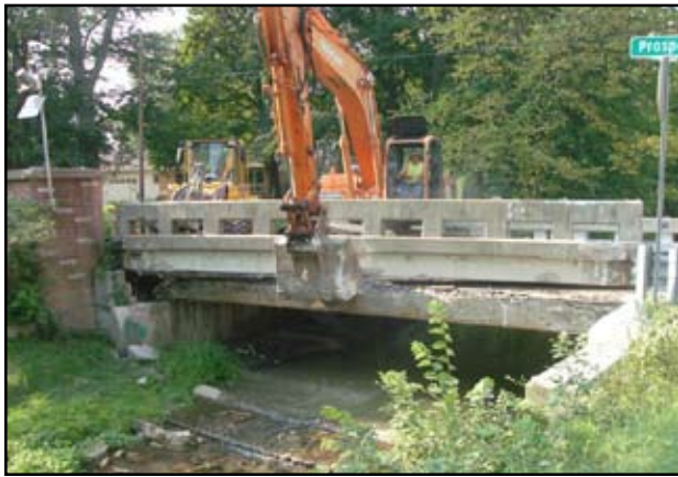
Above, left, construction commences on Prospect Street bridge, which involved removing existing approaches, railing, decking and beams, and constructing all new components. Above, right is the new bridge.
