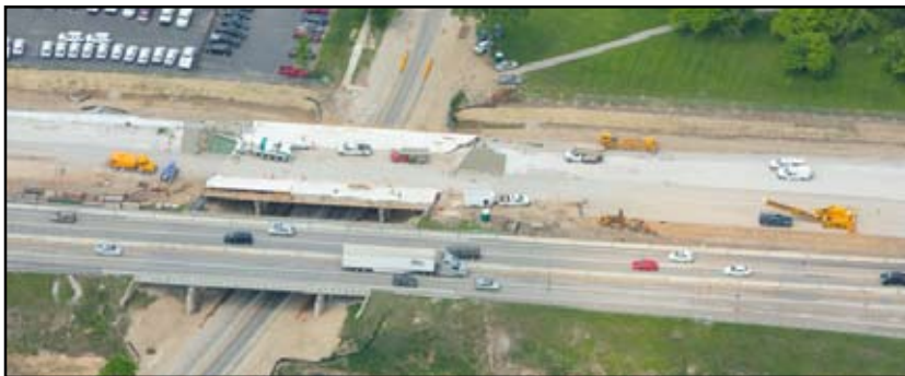
Above is I-69 over Averill Avenue. Existing bridges were widened with micropile-supported foundations. At right is the Dort Highway (M-54) interchange. Complete reconstruction of both overpass structures will allow additional height for vehicles traveling on Dort Highway.
