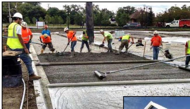
At left, workers from contractor Fessler & Bowman place pervious concrete at the Red Fox Outfitters parking lot. Construction was managed by Rhoads & Johnson. Below is the Red Fox Outfitters building.
