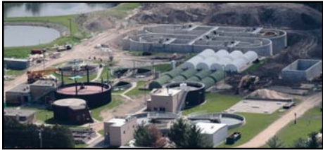
Above is the plant during construction.
