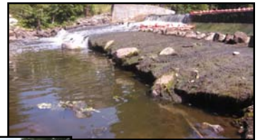
At top, with the absence of water, the undermining of the dam’s concrete spillway apron can be seen during construction. At left is the dam after improvements were completed.
