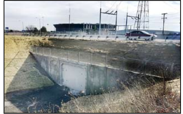
Shown above is the completed project.
