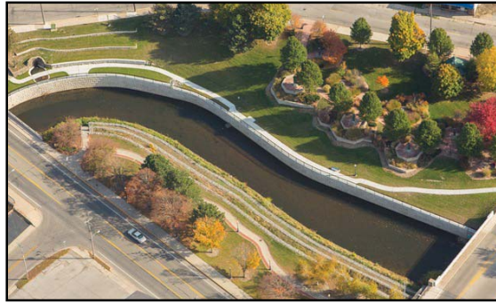
Above, the new wall with the artesian well shown on the left.
