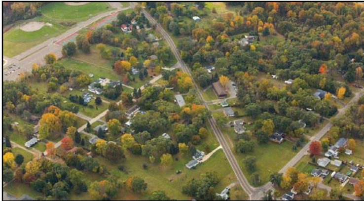
Pictured above is the 0.68-mile completed project.
