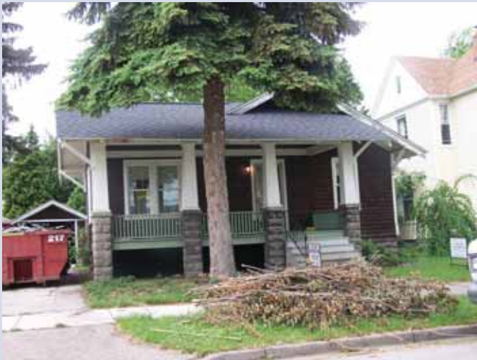
Example of housing rehabilitation in the Presidential Town Center Neighborhood, Bay City, MI.
