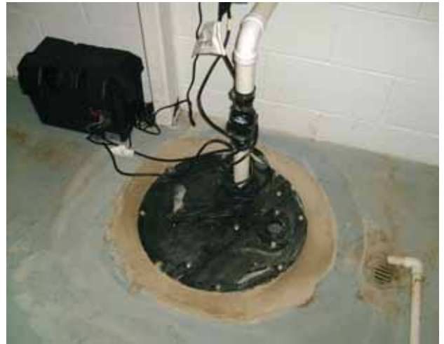
New sump pump installed in Davison, MI home.
