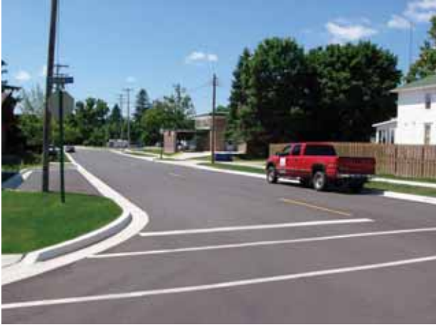
Newly reconstructed 4th Street, Lakeview, MI
