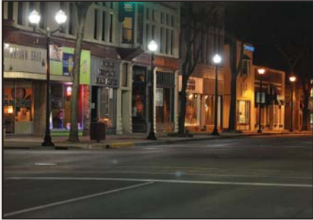
ROWE's project for the City of Alma includes cost-saving LED lighting purchased from a Michigan supplier.
